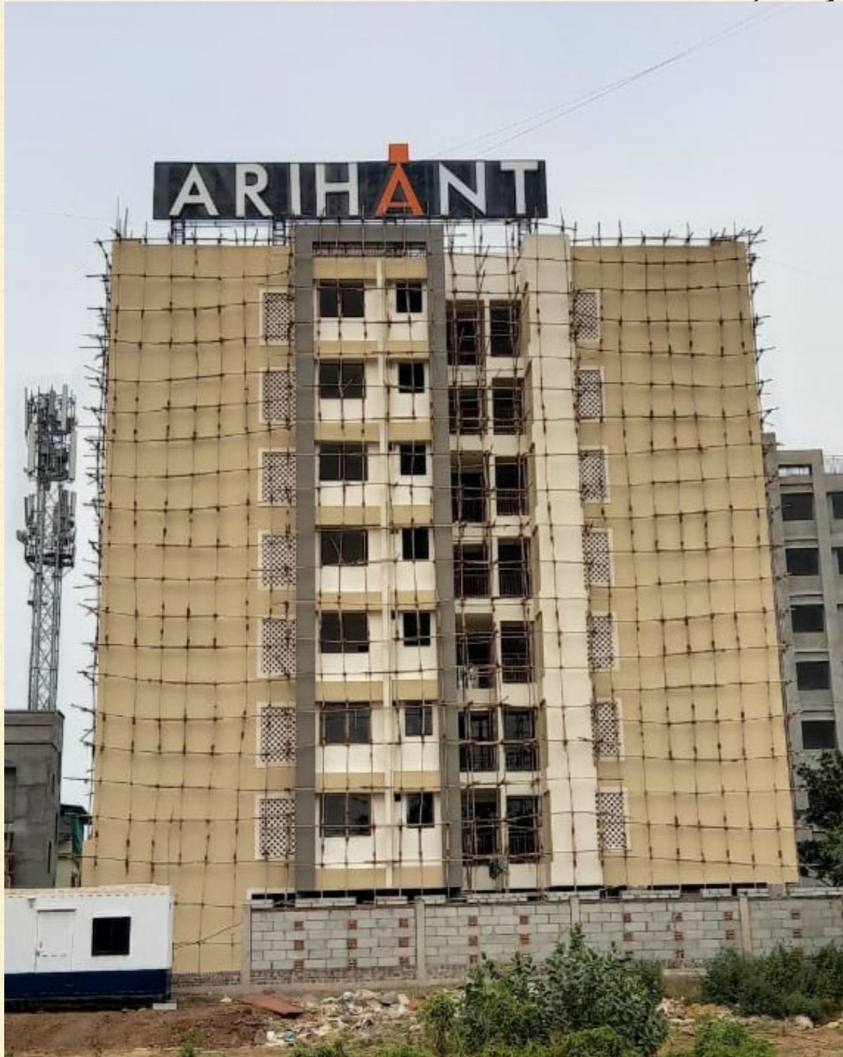
Painting, flooring, firefighting works in progress
