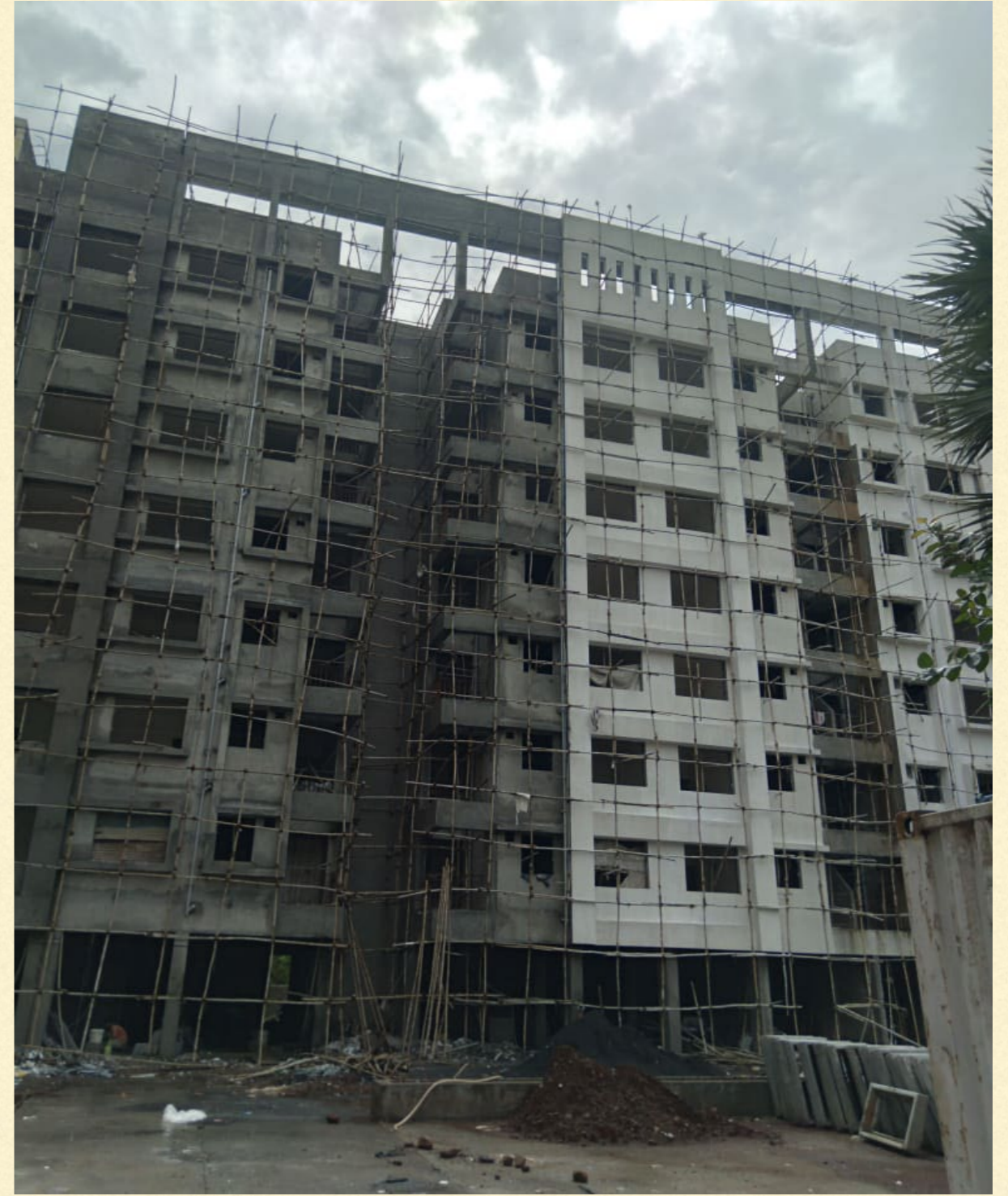
External painting and finishing in progress
