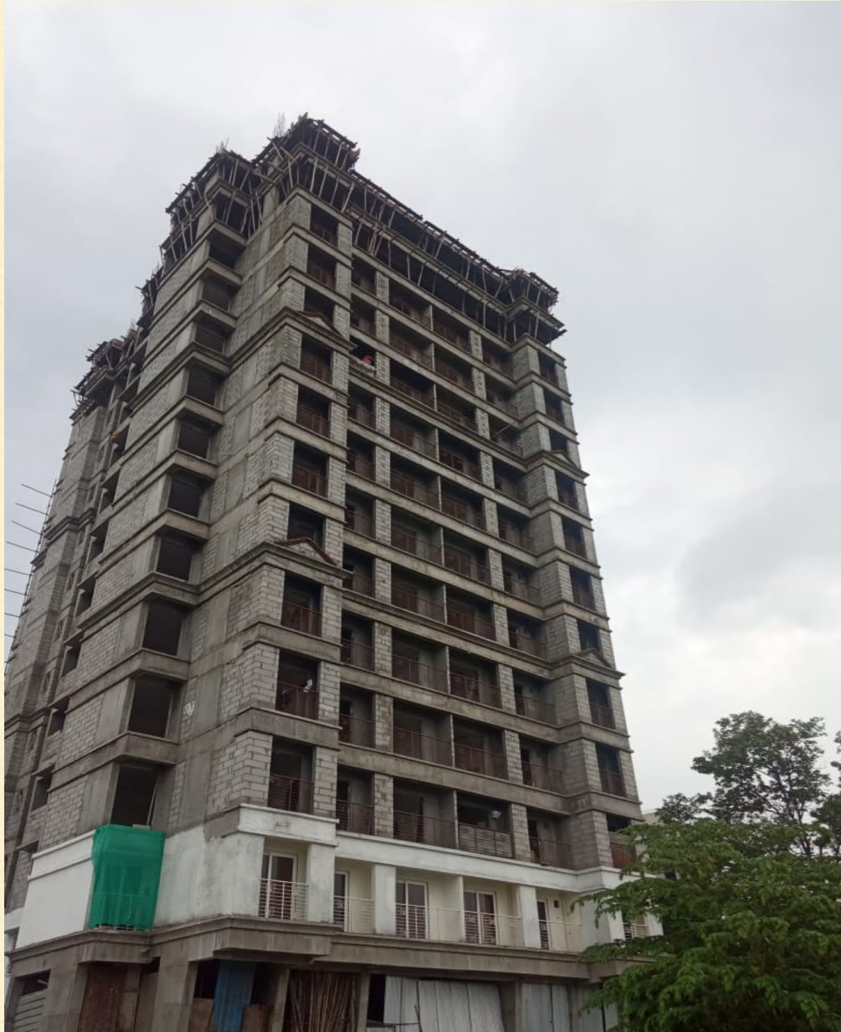
14 th floor completed
