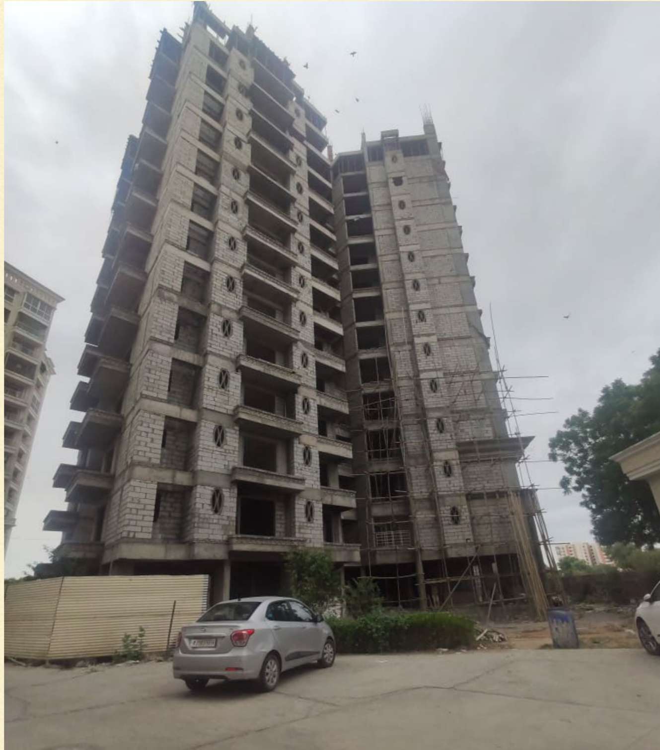
RCC nearing completion & Internal finishing works in progress
