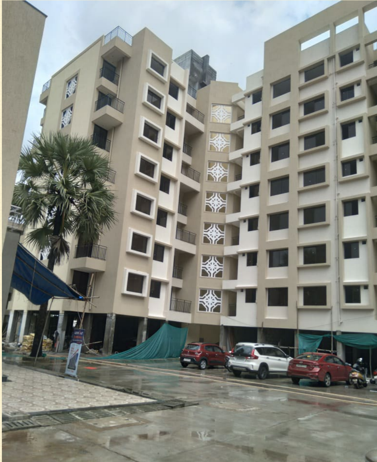
Internal finishing in progress
