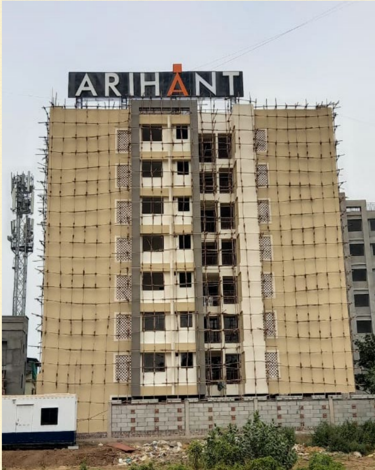
Flooring & Tiling, Doors & Windows completed
