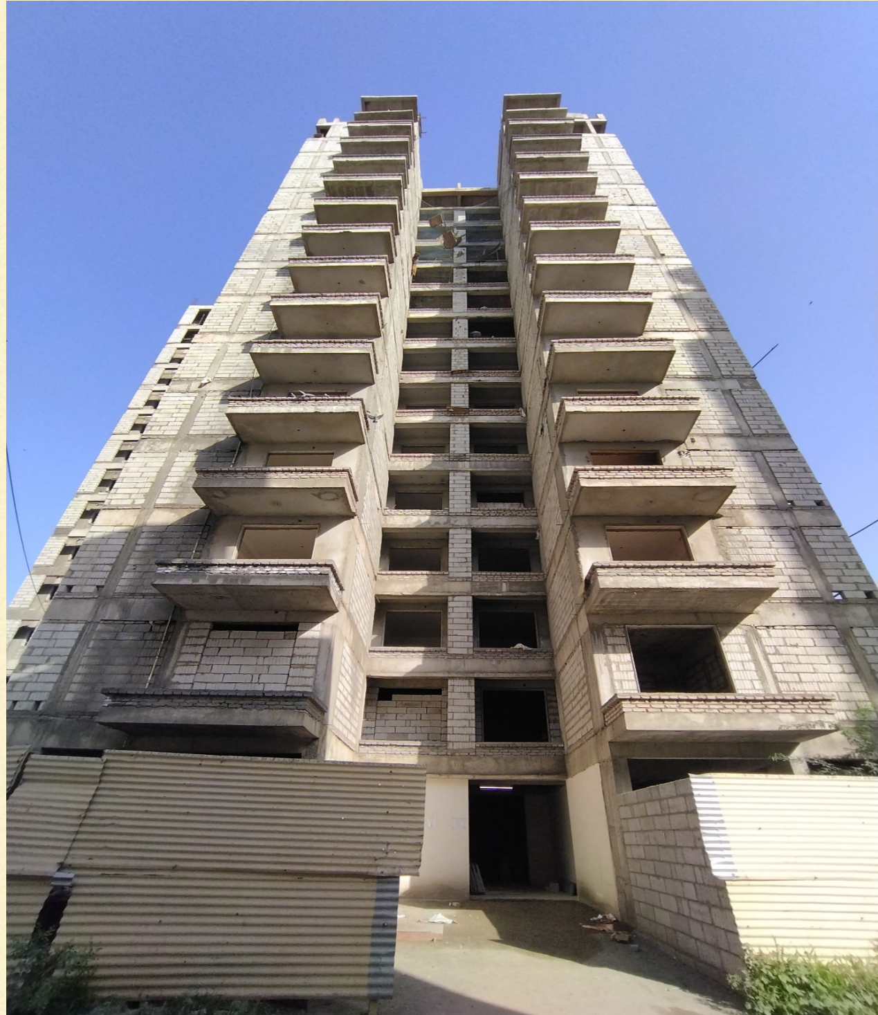
15 th Slab work in progress
