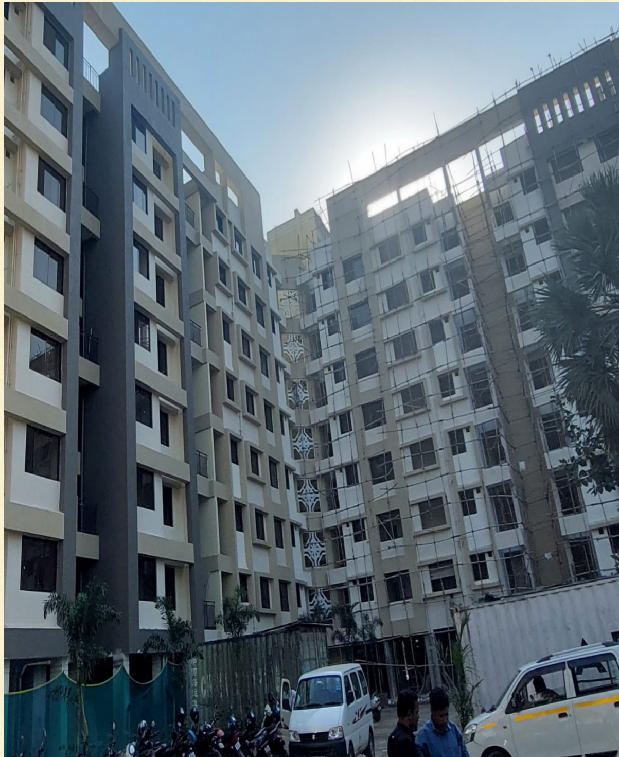
Flooring & Tiling completed
