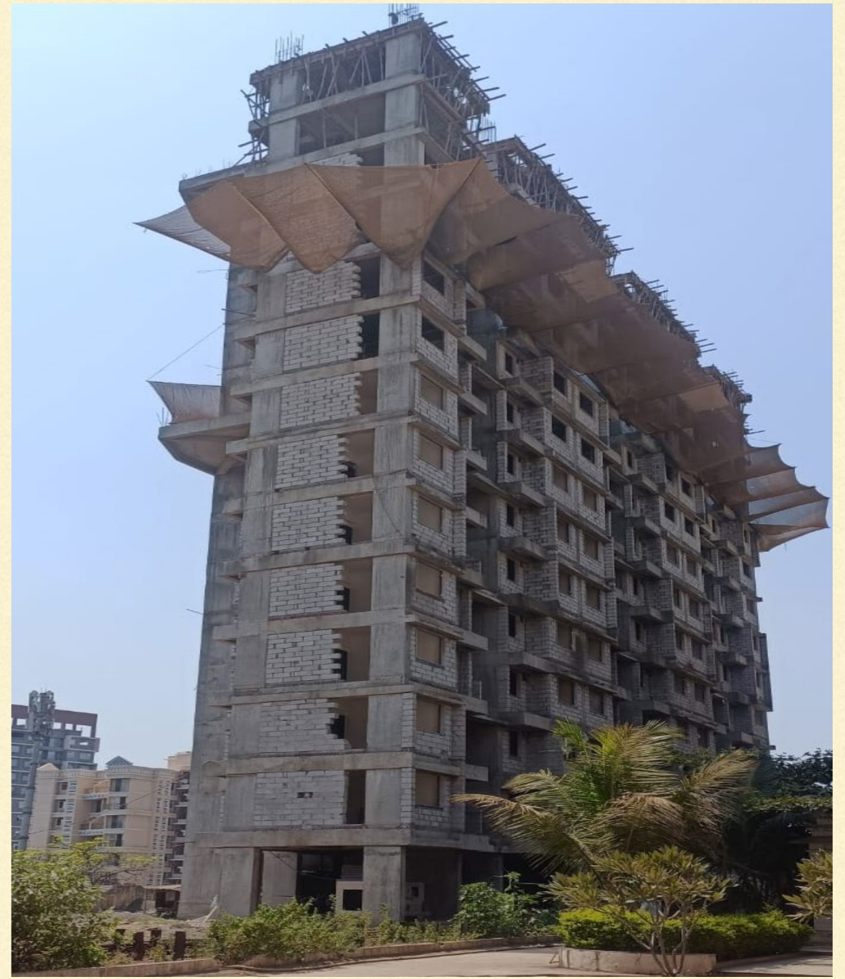
RCC work up to 14 th slab and finishing work till 10 th floor is in progress
