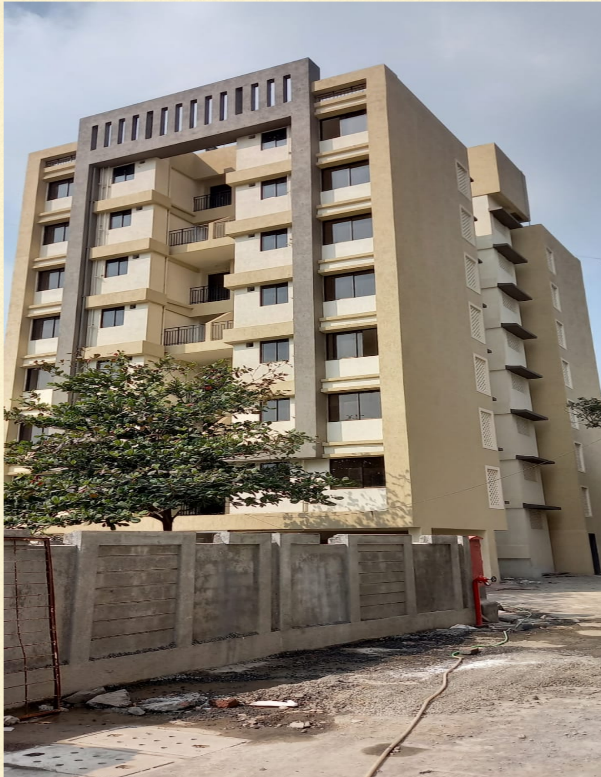
Finishing work nearing completion
